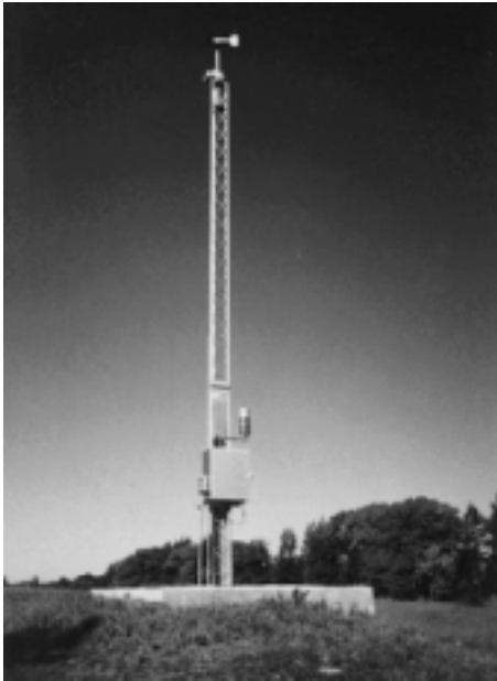
Figure 2: Typical RWIS Tower
